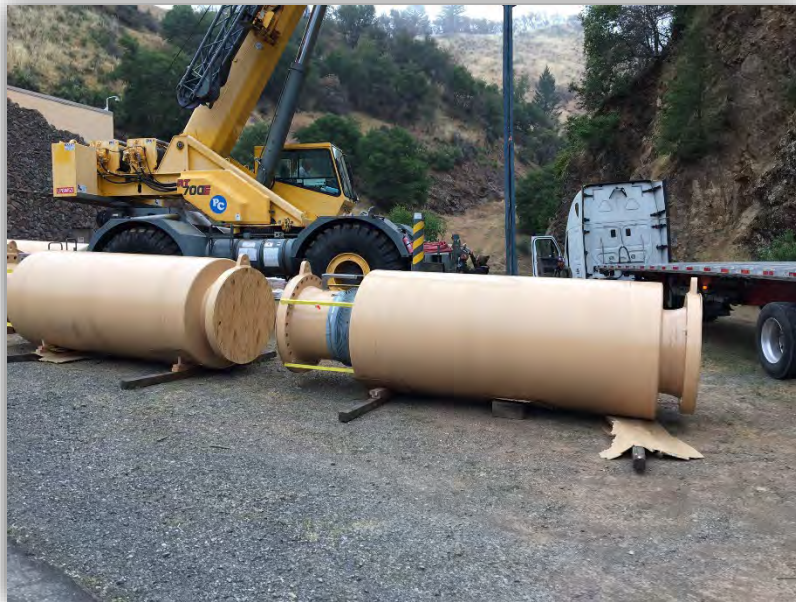
Geysers Pipeline Expansion Joints Replacement
